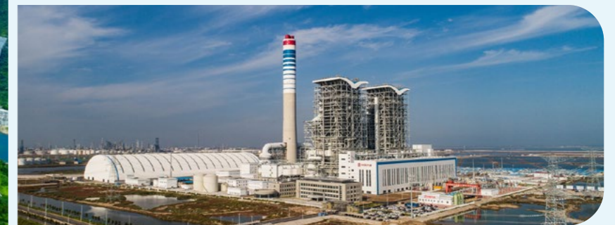
The World's First GW-Level Ultra-Supercritical, Reheated, Six-Cylinder, Six-Row Coal-Fired Power Generation Unit — CDT Dongying No.1 Power Plant Unit
