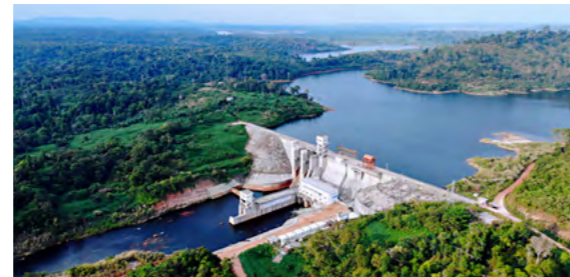
Cambodia Stung Atay Hydropower Project
