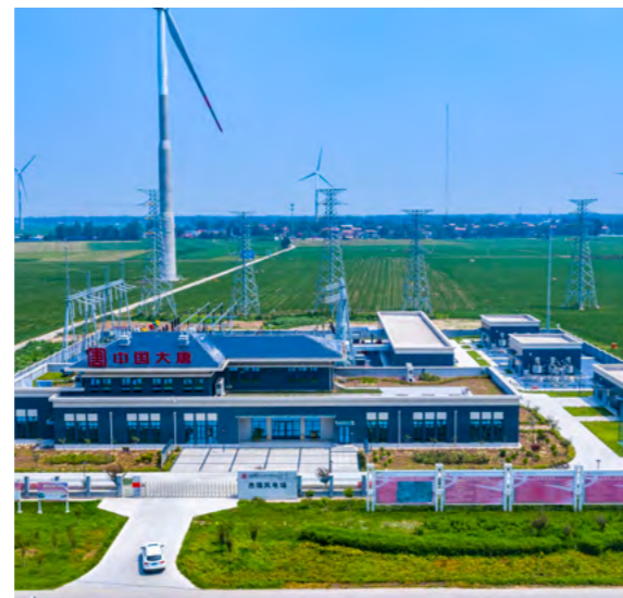
Zaocun Wind Farm Project in Huaxian County, Henan Province, won "the 2022 China Electric Power Quality Engineering Award", the highest honor of engineering quality in the power construction industry
