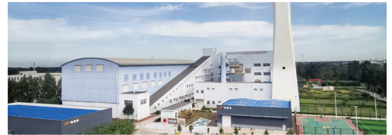
Datang Baoding Heat Supplying Co. Ltd.
