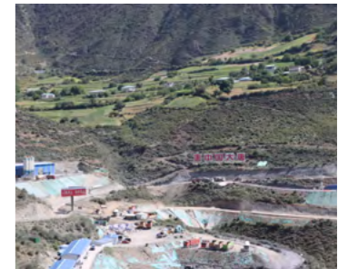
Construction Site of Zara Hydropower Station
