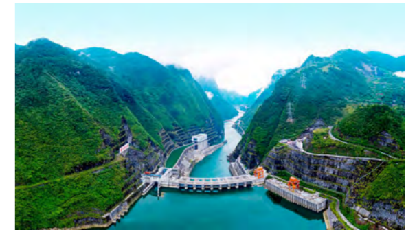
Dam of Pengshui Hydropower Plant
