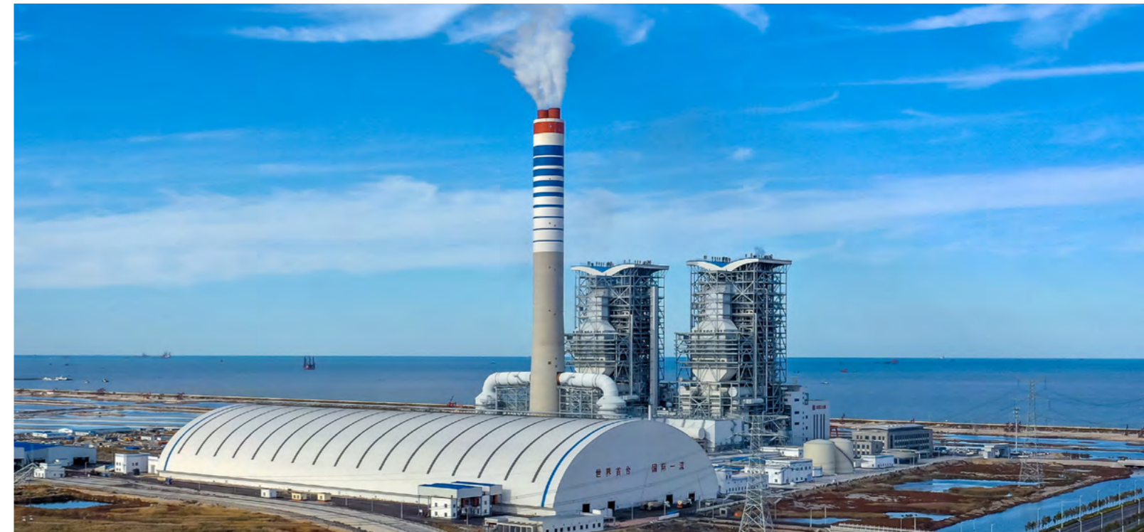
On November 14, 2022, No. 2 Unit of Datang Dongying Power Generation Co., Ltd. successfully applied the intelligent startup and shutdown system to complete the one-click grid connection, which is the first 1 million kW unit to realize whole-process intelligent start until load-carrying status in the Group.
