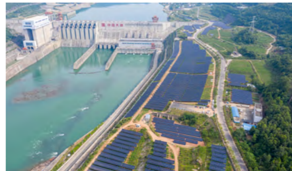
Tingzikou Water Conservancy Hydro-junction Project is the only control project on trunk stream of the Jialing River, which is known as "the Dujiangyan Irrigation System in the New Era"
