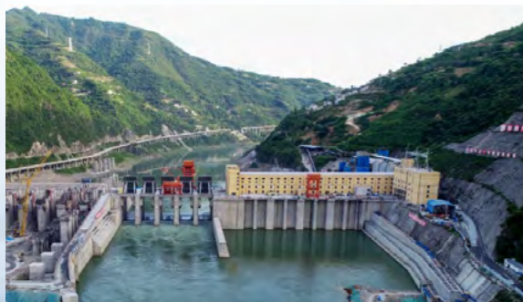
In December 2022, four units of Xunyang Hydropower Power Plant underwent 72-hour test-run, setting a new record of "putting four hydropower units in operation within a single month" for the Hanjiang River Basin in Shaanxi Province
